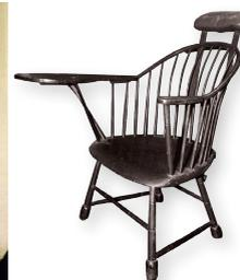
American dentist, constructs the first chair made specifically for dental patients. He does so by attaching an adjustable headrest, plus an arm extension to hold instruments, to a wooden Windsor chair.
